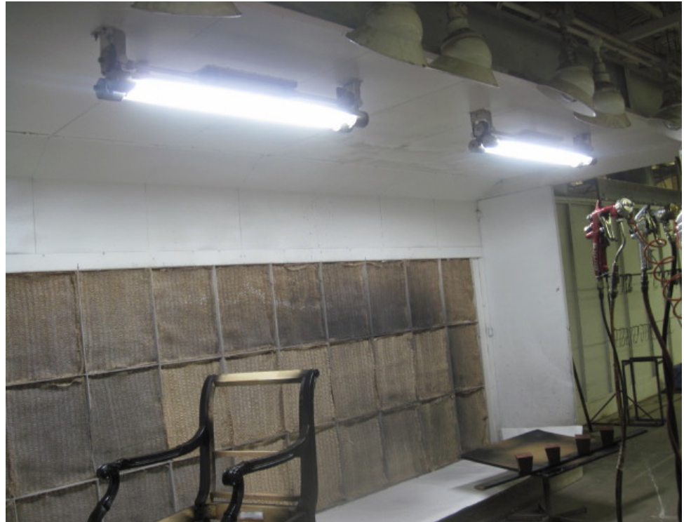
Old fluorescent lighting was replaced with high efficiency lighting in the spray booths, which also increased the quality of the light for workers performing that function.
