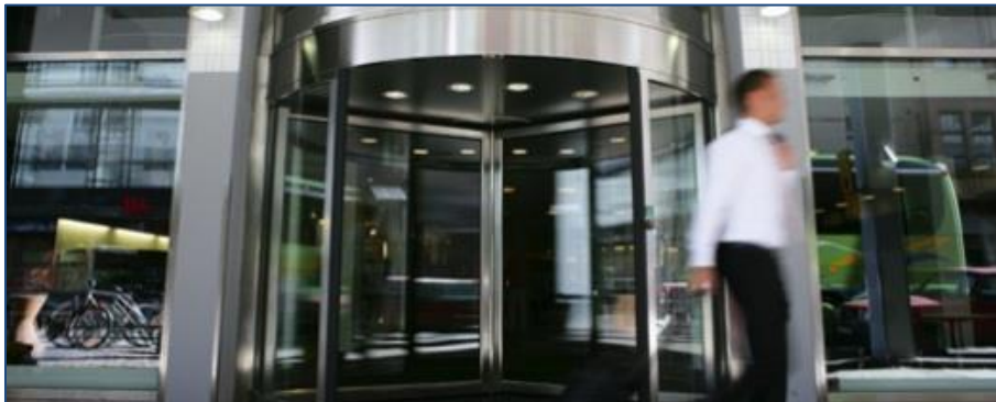
Besam North America/Assa Abloy saves energy through collaboration with the NC State University IAC and E3 Programs. Photo courtesy of Besam.
